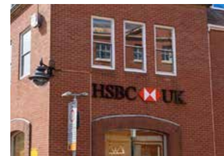
Lighting - Building mounted
