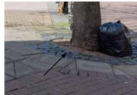
Tree Pit - Basalt setts circle
