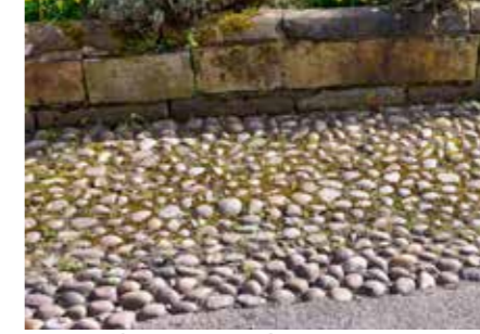
Back of paving/infill - Cobble on edge detail
