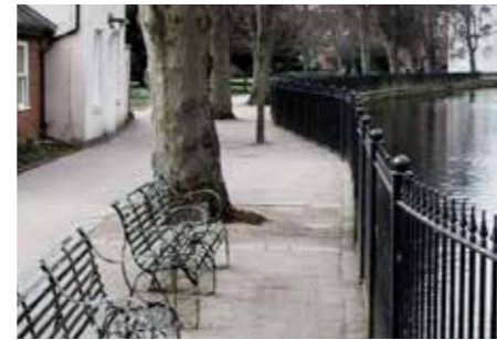
Tree pit - Asphalt with concrete flag surrounds
