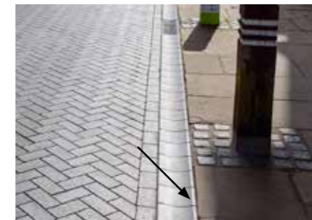
Channel - Blue eng brick (running)
