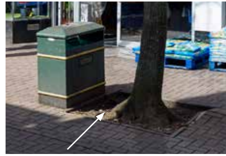
Tree Pit - Square, concrete pin kerbs
