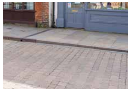
Highway - Concrete tegula paving multi
