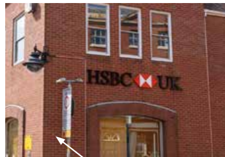
Lighting - Building mounted
