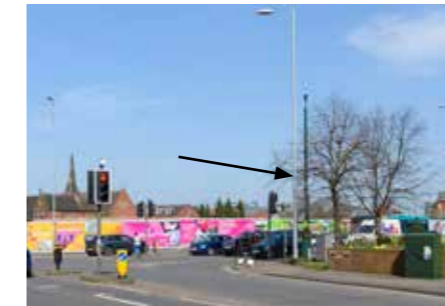
Lighting - 10m highway lighting columns
