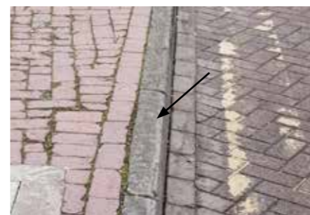
Kerbs - St John's transitions to full height concrete
