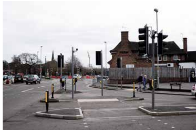
Vehicle and road infrastructure dominate Greenhill
