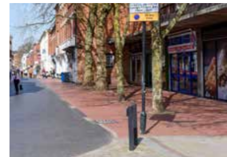
Footpaths - Red brick (stretcher) to arcade
