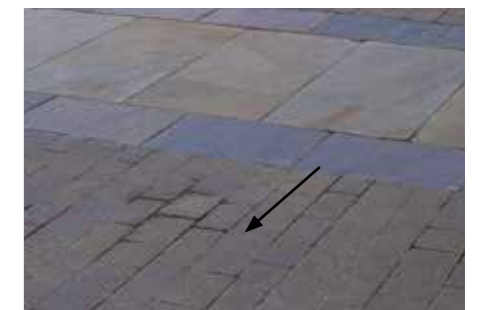
Paving - Buff multi concrete pavours
