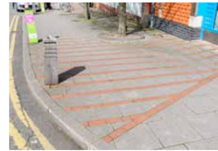
Footpaths - 400 x 400 concrete slabs, red brick banding detail
