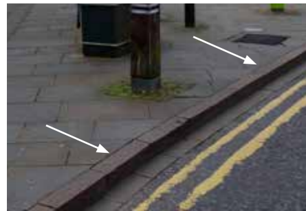
Kerbs - Red granite transitions from 75-150mm high
