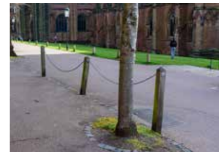
Bollards - Square timber with chain
