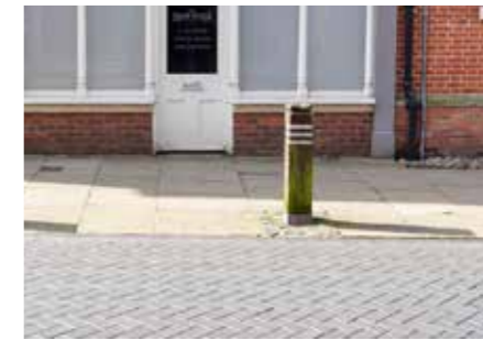
Bollards - Square timber
