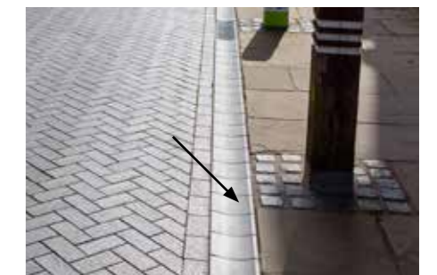
Channel - Blue eng brick (running)
