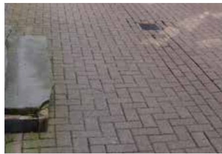
Highway - Buff concrete pavours (herringbone)
