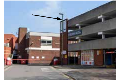
Lighting - Highways lighting columns
