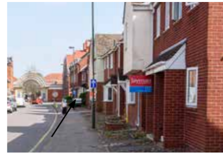
Lighting - Highways lighting columns
