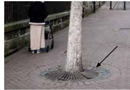
Tree Pit - Circular steel grilles
