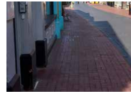
Footpath - Red eng brick (basket weave)
