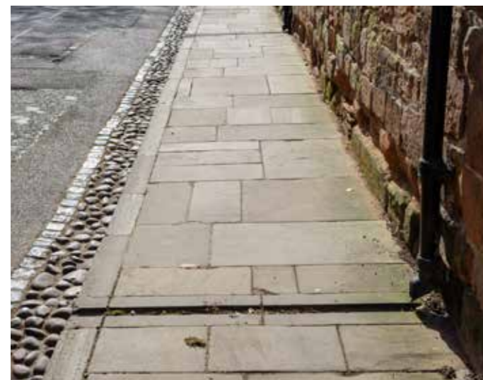
Cut stone drainage channel within pavement - Cathedral Close
