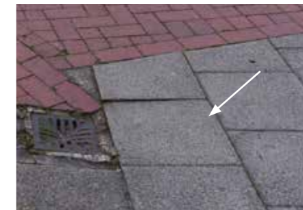
Footpaths - PCC flags to south west
