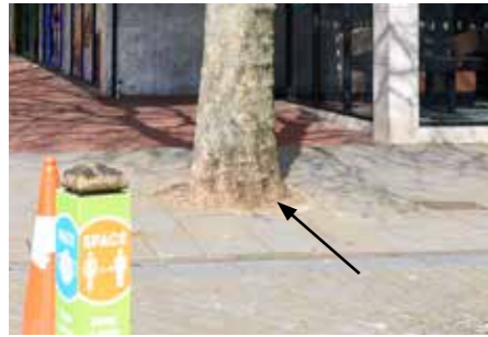
Tree Pit - Circular basalt sett trim
