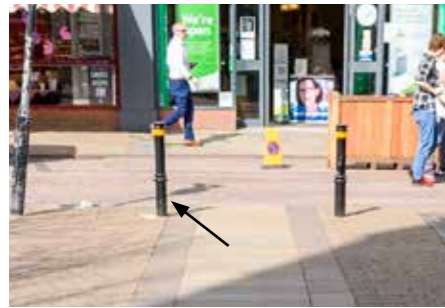
Bollards - Contemporary black steel, fluorescent band to top
