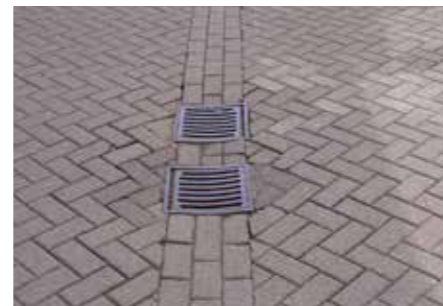
Channel - Concrete paviours (stretcher) central
