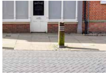
Bollards - Square timber
