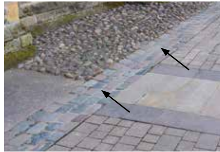
Channel - Multi rectangular granite setts
