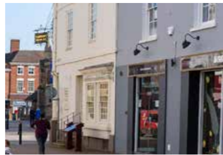
Lighting - Building mounted
