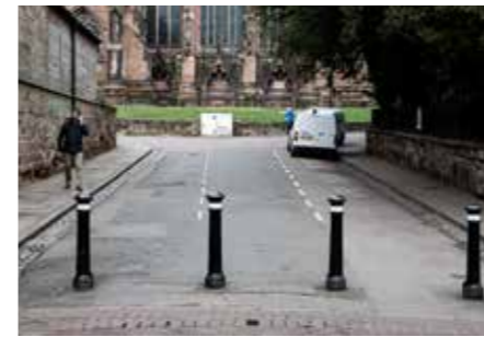
Bollards - Heritage black steel vehicular bollards
